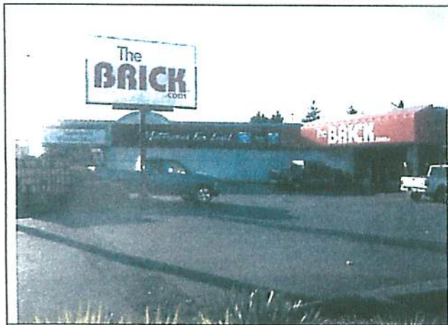
Exterior fronting South Fraser Way
