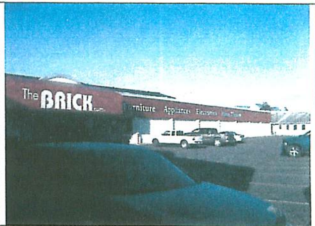
Exterior fronting South Fraser Way
